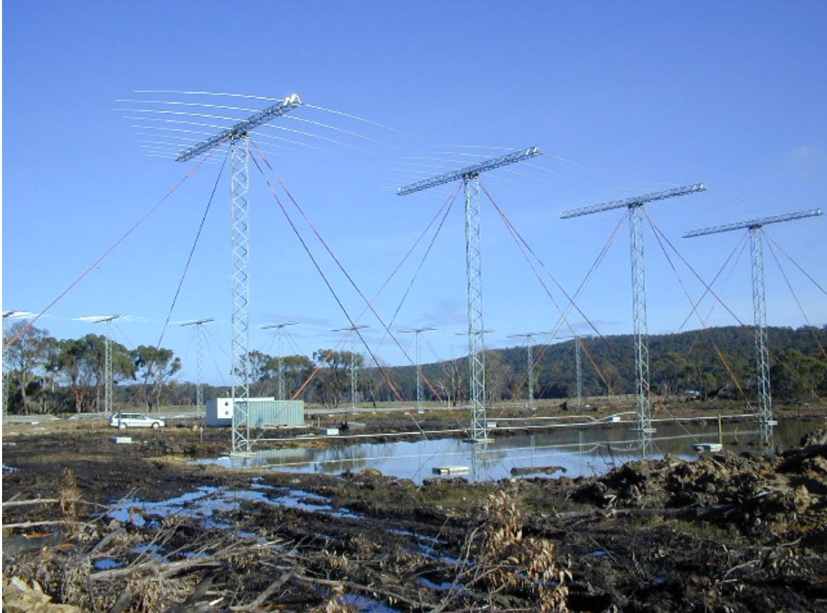
Figure 1.1: The TIGER Bruny Island radar viewed from behind. The 4 antenna interferometer array is shown in the foreground and the 16 antenna main array in the background.
