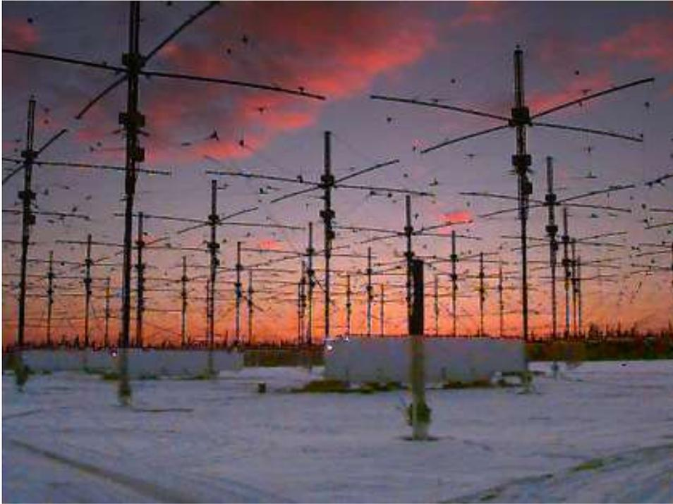
Figure 1.5: The HAARP Ionospheric Heater near Gakona, Alaska. The phased array crossed dipole antennas are clearly visible. From: <http://www.haarp.alaska.edu>
