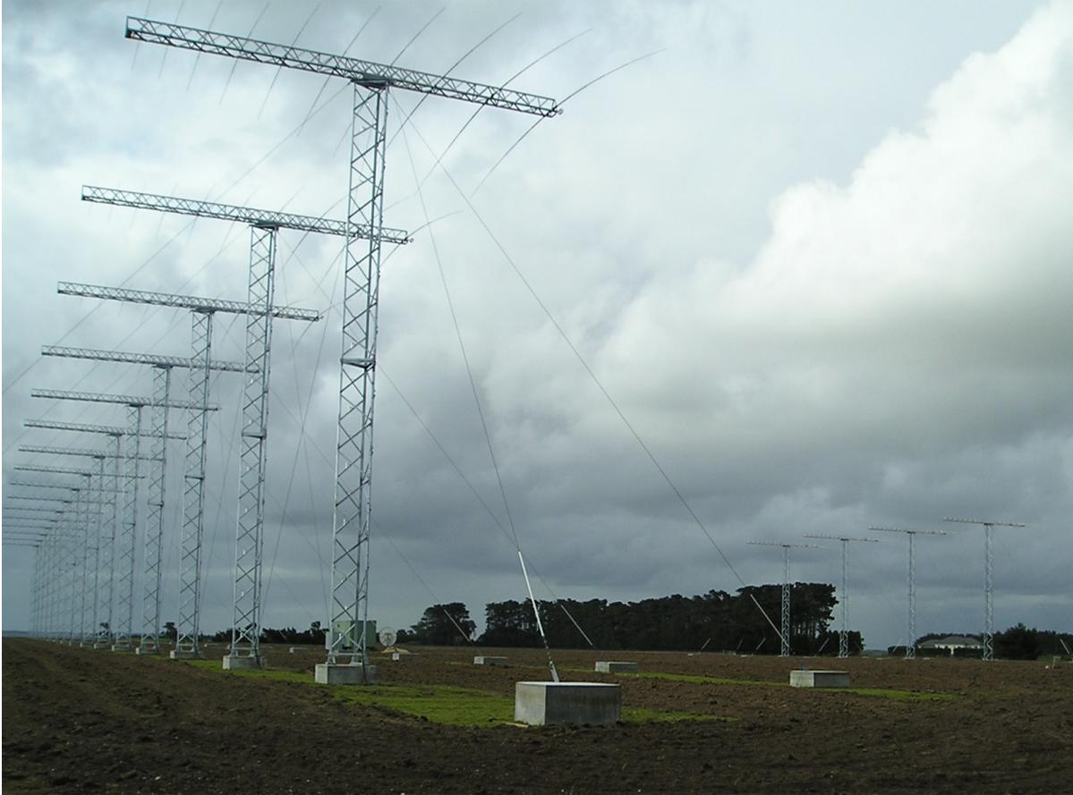
Figure 1.2: The TIGER Unwin radar viewed from the front. The 16 antenna main array is shown in the foreground and the 4 antenna interferometer array in the background.
