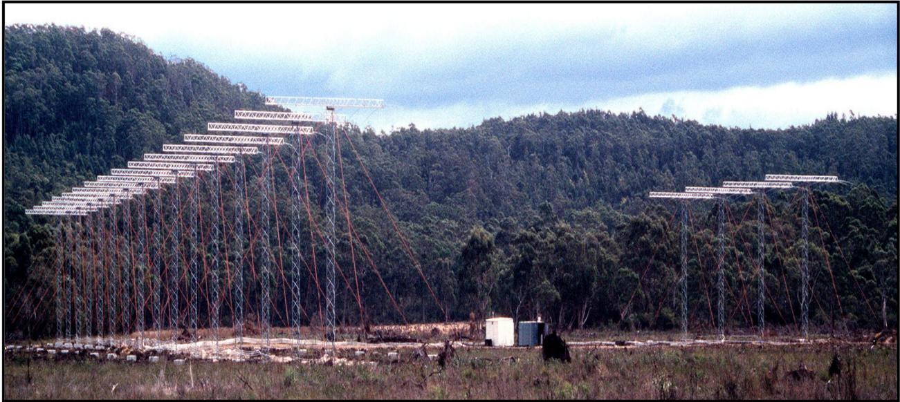
Figure 2.3: The 16 log-periodic elements of the TIGER radar and its 4 element sub-array (courtesy of Danny Ratcliffe).
