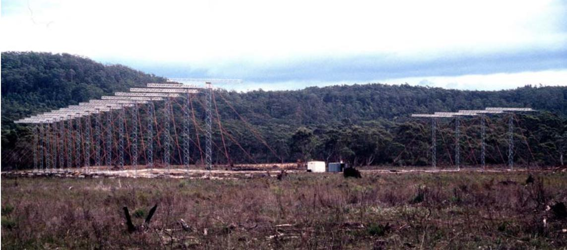
**Figure 2.1:** The TIGER radar consisting of 16 transmitting and receiving antennas in the main array and 4 receiving only antennas for the interferometer sub-array (courtesy of Danny Ratcliffe, Australian Antarctic Division).
